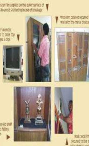
Polyester film applied on the outer surface of glass to avoid shattering in case of breakage
