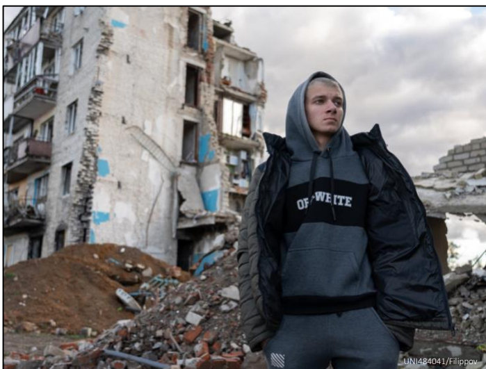
Figure 2: 17-year-old Habriel is standing in front of a building, destroyed by the shelling on 28 October 2023 in Izium, Ukraine.
