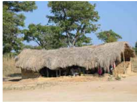
Image 2: a rural school with a thatched roof and no walls constructed by villagers
