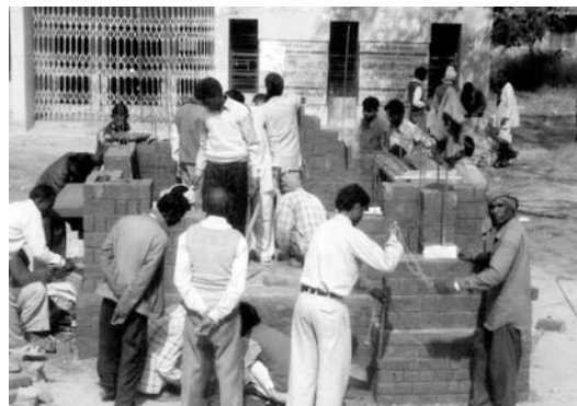
Figure 14: Masons learning hazard resilient building practices in Uttar Pradesh
