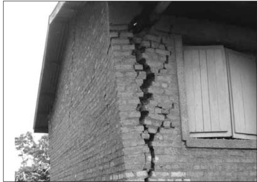
Figure 8: Earthquake induced cracking on this school in Rwanda
