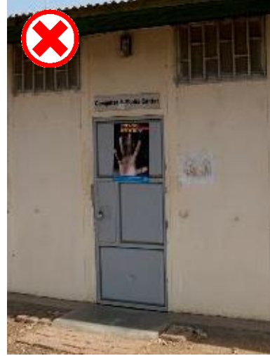
Poor accessibility to the computer room entrance, Malawi 2014 © Sandrine Bohan-Jacquot
