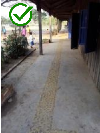
Tactile (pebble) strips for guidance © HI Cambodia 2012
