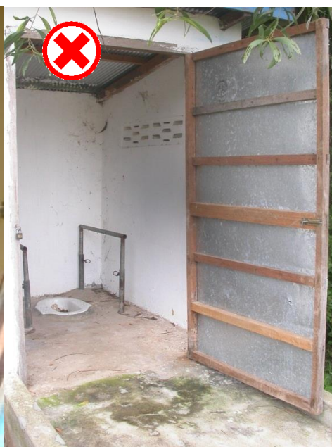
Jones and Reed (2005) - a chair with a hole should be added to make the toilet accessible
